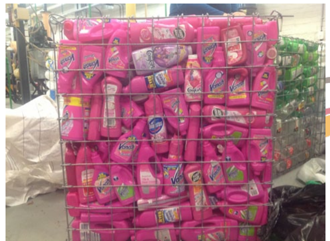
Filling of the gabions with recycled waste from Masiphumelele and Interwaste.
